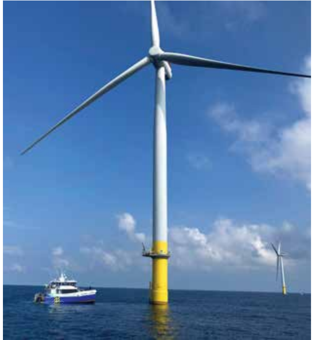
CTV Atlantic Endeavor at WTGs. Picture source: Dominion Energy.
