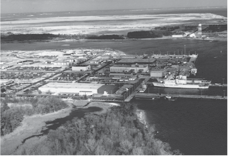
Coast Guard Base Support Unit, Portsmouth, Virginia.
