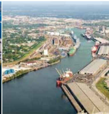
Port of Houston Authority Project 11 Ship Channel Expansion.
