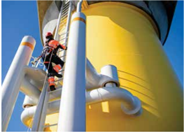
Technician Working on Turbine. Picture source: Ørsted.
